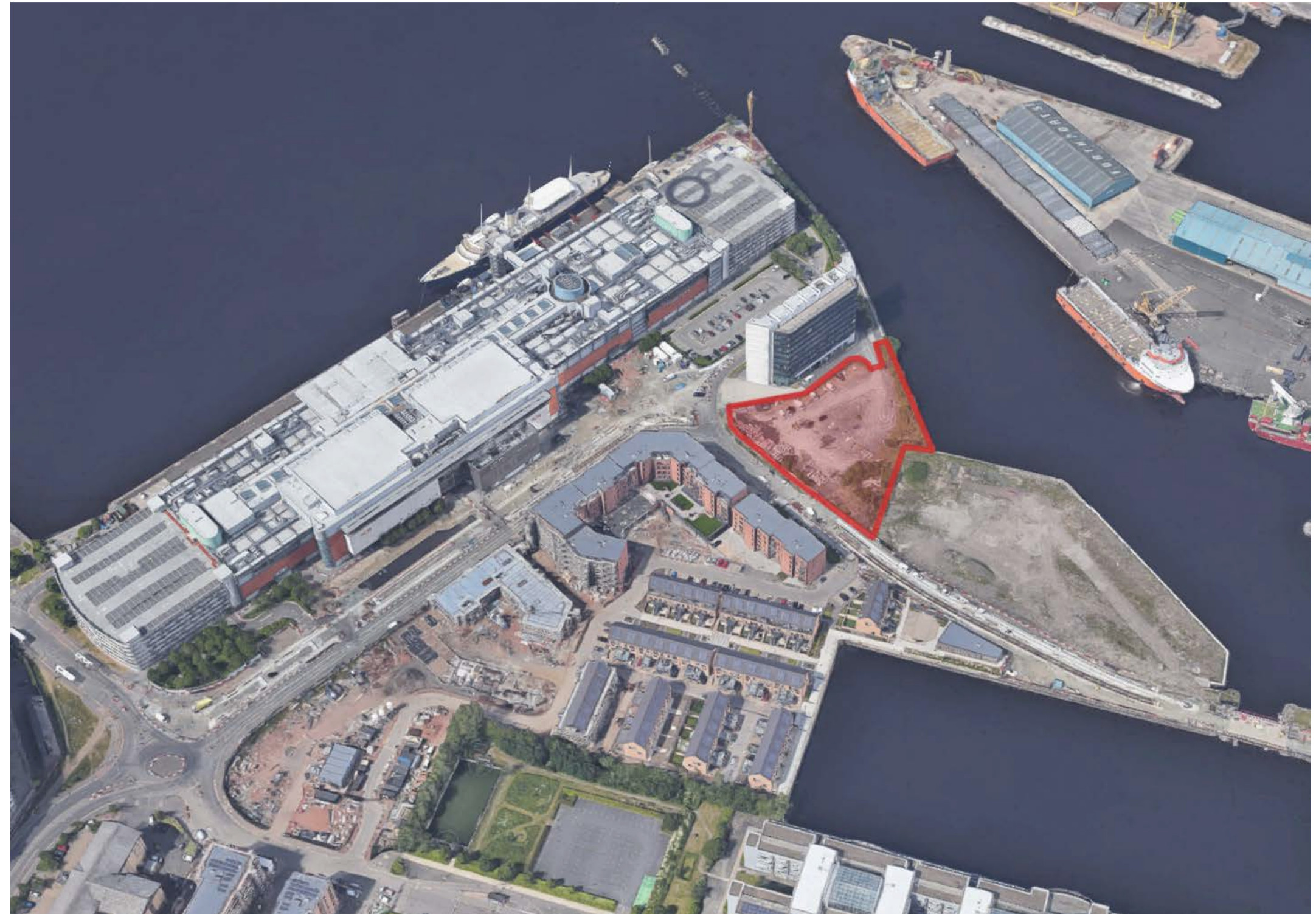
Ocean Drive site looking north west
